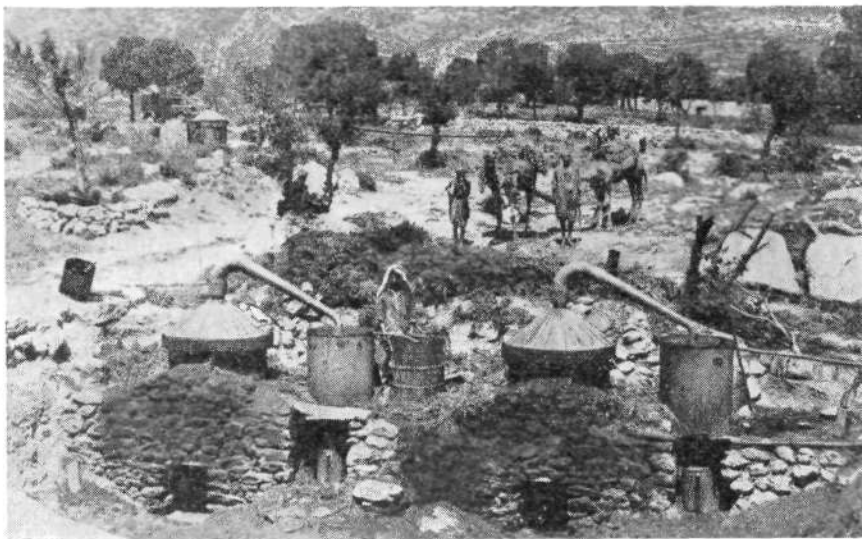
PLATE 4. Field distillation of rosemary in Tunisia. The stills are directly fired. The plant material is transported by camels to the distillation post.
